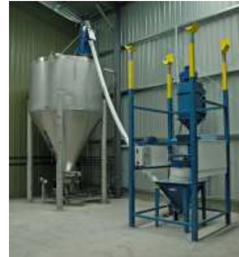
with forklift loading
